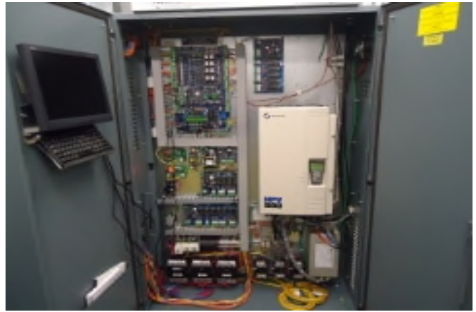
All four elevators and cabs were recently renovated to improve performance and meet current code requirements.
