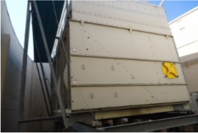
Cooling towers are performing without major problems.
