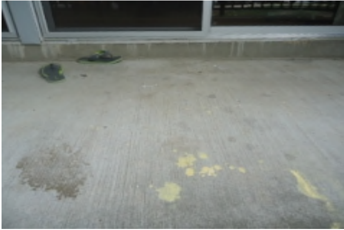
Sealer placed on balconies years ago to prevent concrete structural damage has worn thin. Sealer reapplication should be done within the next two years.
