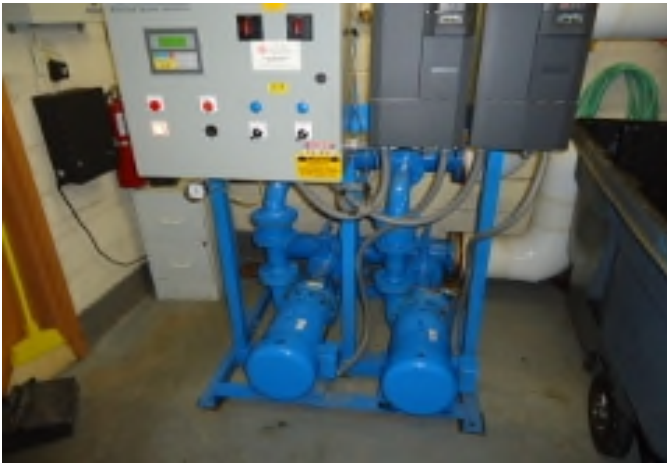
Water booster pump was recently replaced.
