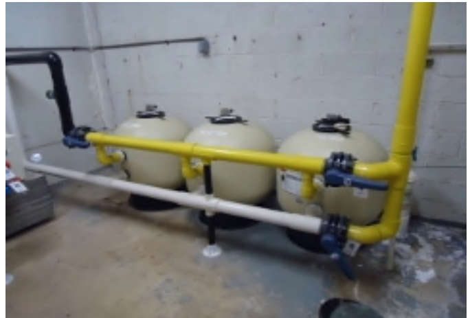
Swimming pool to include shell, deck, filters, water heaters, handicap bathroom and fence were all recently re-furbished.
