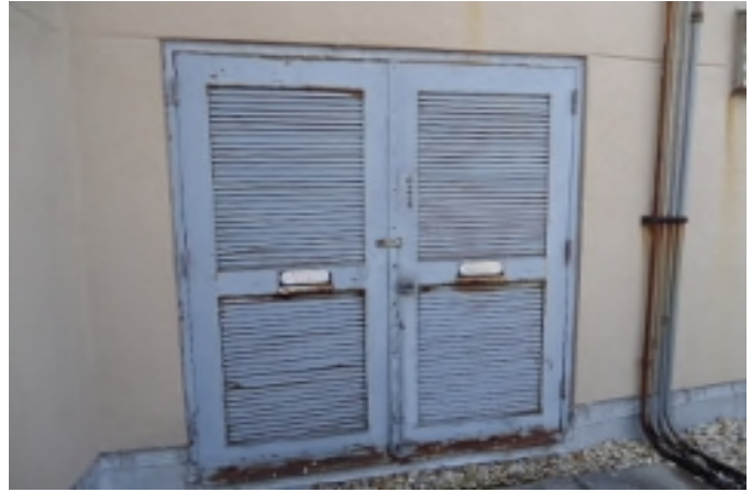
Entrance door to roof-top mechanical room is corroding. Periodic painting will control rust and extend the doors useful life.
