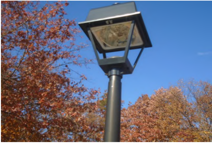
Typical street light - reserve entry does not assume all units will be replaced at once but rather spot repairs to posts, fixtures, ballasts, sensors, etc. will be made as needed.
