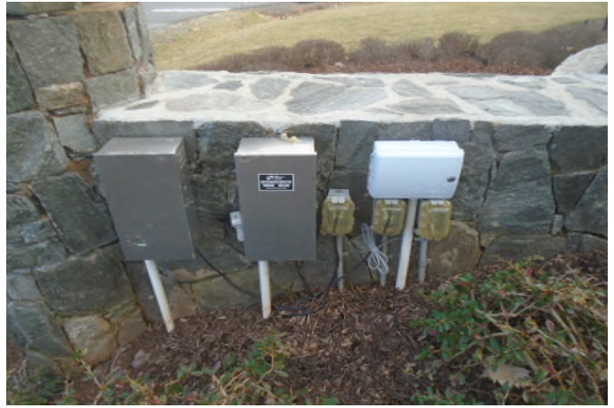
Electric service to entrance feature flood lights, wiring and electric panels are reserve components. As is upkeep of the irrigation system that can be kept in good repair with spot repairs.
