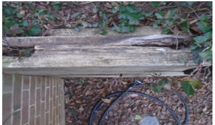
Typical of retaining walls - top rail usually deteriorate. Rest of the wall is structurally sound - replacing top rail will extend the walls useful life.
