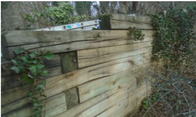
When retaining wall total replacement is needed consider installing a modular block (segmented) system. These systems have a longer useful life and require less maintenance.
