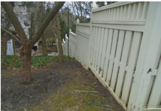
Useful life of fencing can be extended by painting/staining, nailing or screw fastening warped boards, straightening and doing other repairs, as needed.
